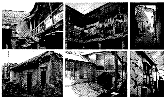
Fig. 2 Different exterior view of conventillos' physical condition
