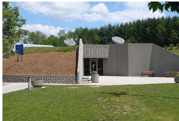
Fig. 2.3. Earth sheltered rest area along Interstate 77 in Ohio.
