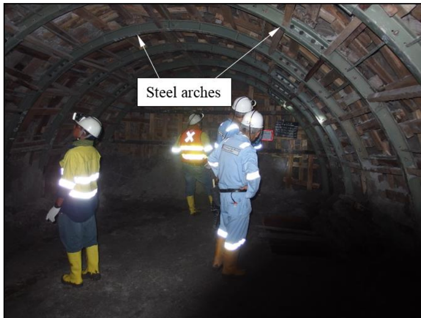
Figure 2.9 Steel arch support installed in main roadway at GDM coal mine.
