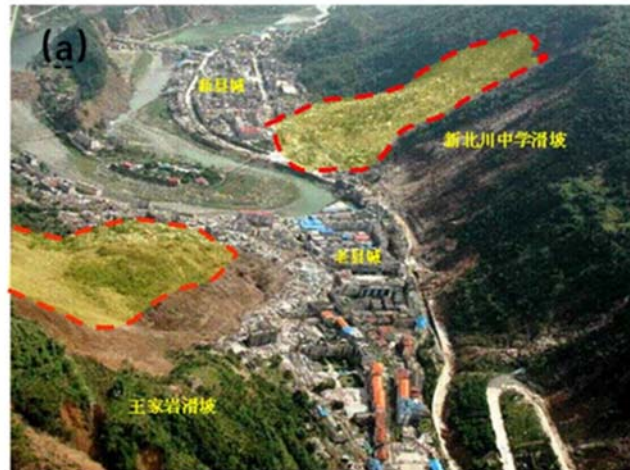
Figure 1-2 Image of the New Beichuan Middle School landslide induced by the 2008 Wenchuan Earthquake, China. Source from NASA .
