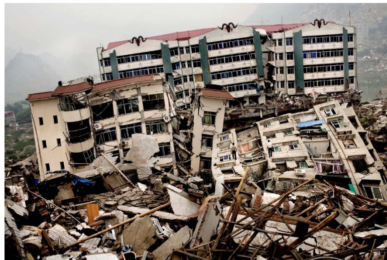
Figure 1-3 Image of collapsed buildings during 2008 Wenchuan China earthquake. (access from internet)
