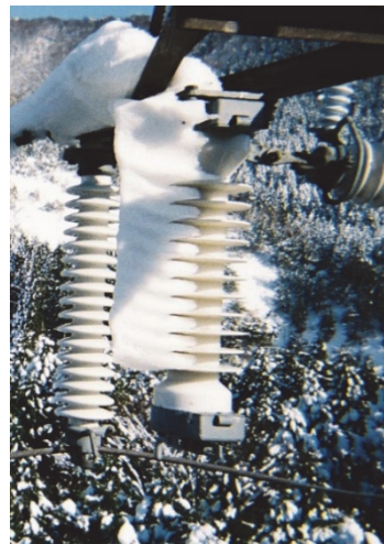
(b) Lightning arrester assembly
