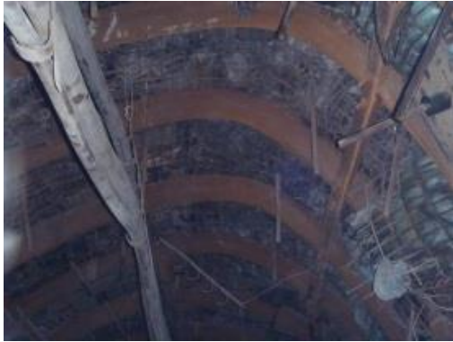
(a) Steel arch shed
