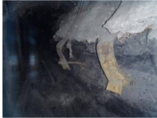
(b) Conventional rock bolt
