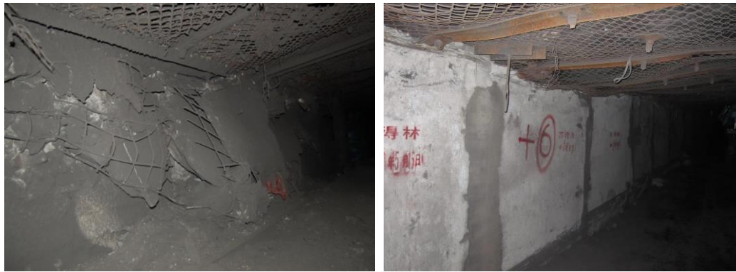
(a) Before roof pre-split
