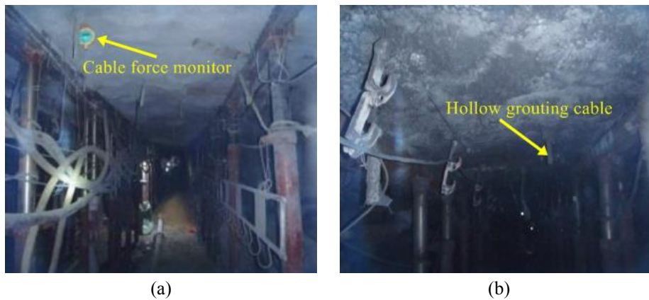
Fig. 5-17 Profiles of the RGSG 100 m behind the mining face
