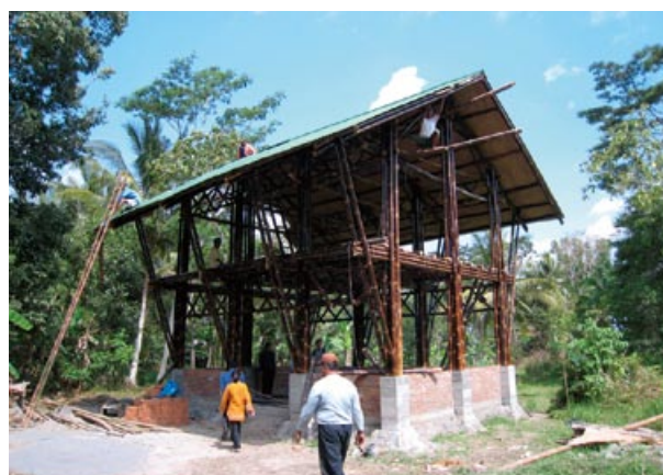
Fig. 3 Two stories local house under construction. Bamboo is used as construction material that is research output by Prof. Munawar group of Civil Engineering Department.
