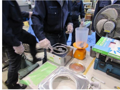
(f) Epoxy putty measurement (1600gr/m 2 )
