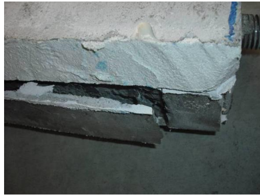
(b) The feature of failure
