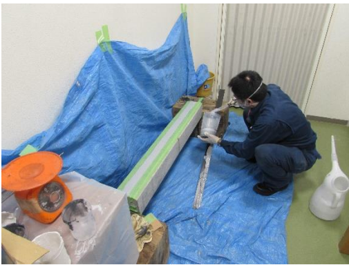
(g) Epoxy putty application (treatment \pm 2days)
