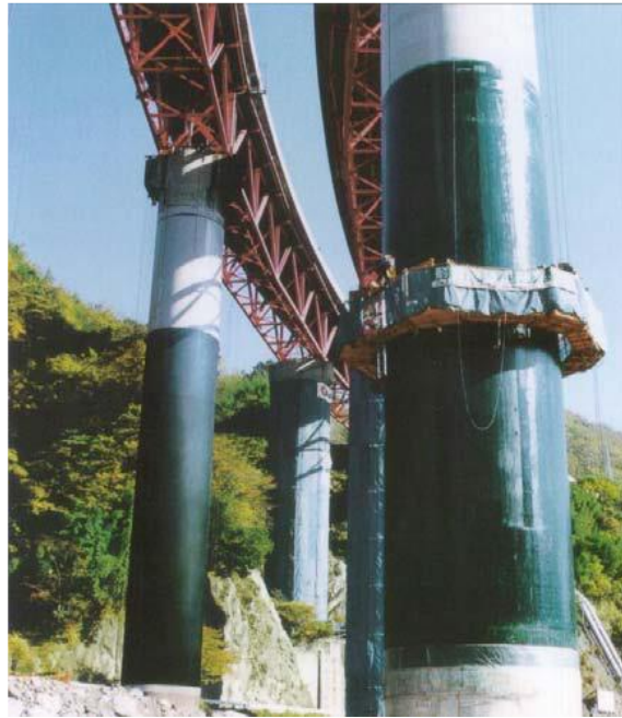
Photo 2.5 Seismic retrofitting of high piers (2.12)
