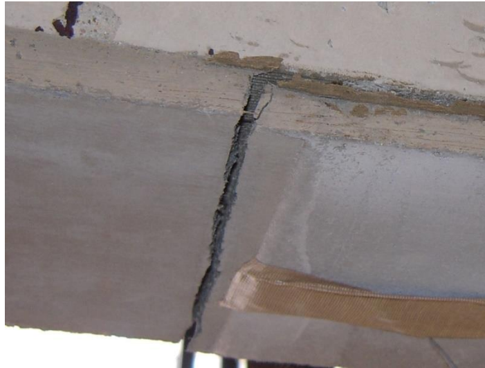
Photo 3.3 Failure detail of specimen PCM2
