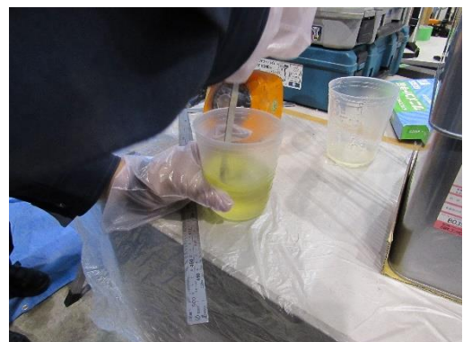
(b) Epoxy resin primer measurement (200gr/m 2 )
