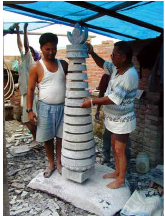
Figure 4. Nepalese stonemasons checking the fit of pre-carved components for the uppermost section of the stupa in Kathmandu, Nepal. Photograph by Holm Triesch, 2003.
