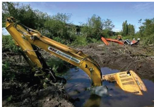
Figure 3.30: On site difficulty in peat stabilization
