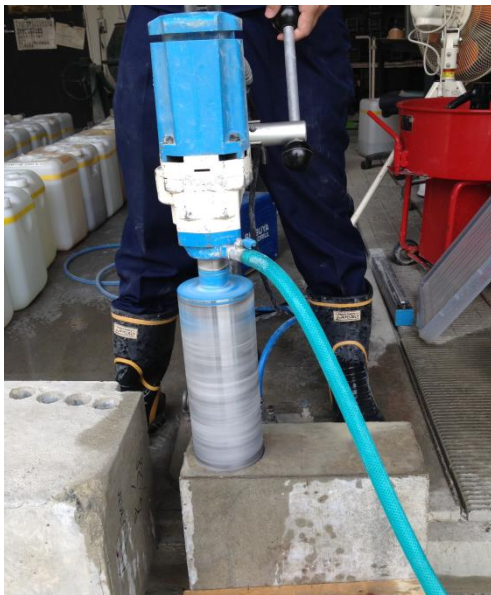
(a) Core drill of mortar sample
