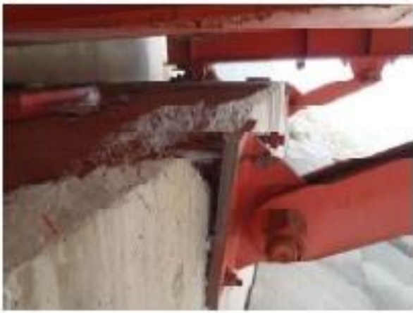
(a) Bridge restrainer system (Munemoto and Sonoda, 2012)
