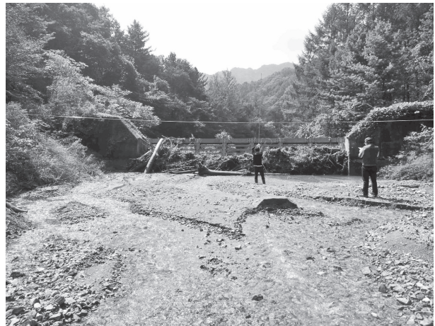
Fig. 2. LWD trapped by buttress check dam at the outlet of the catchment (16 September 2013).
