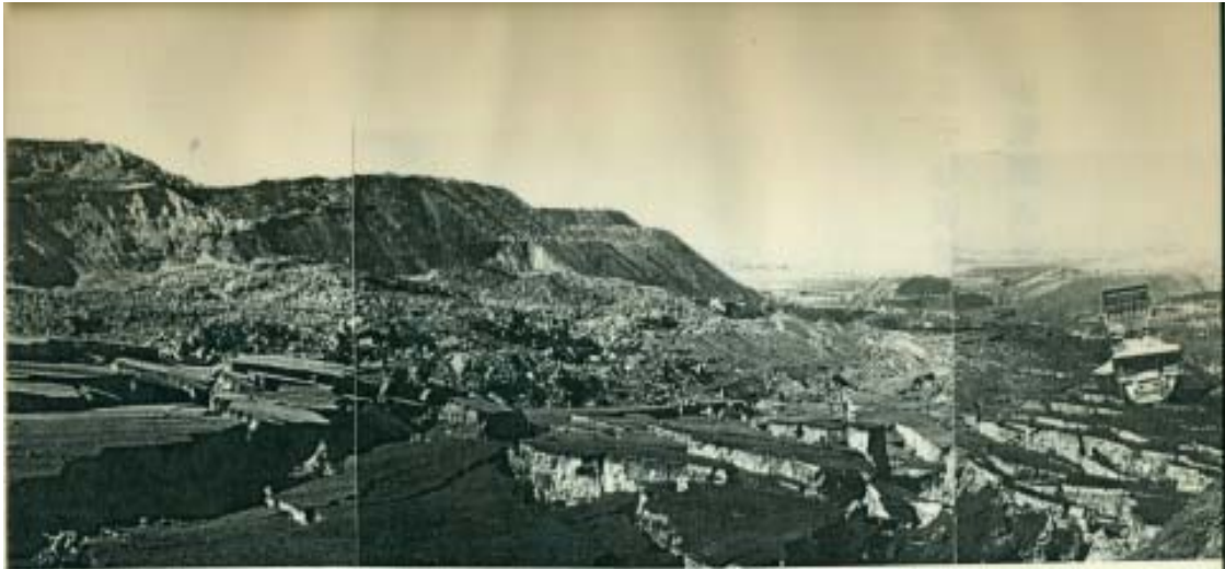
Figure 2.1 Slide of the dumping area and the trucks were trapped in the sliding mass
