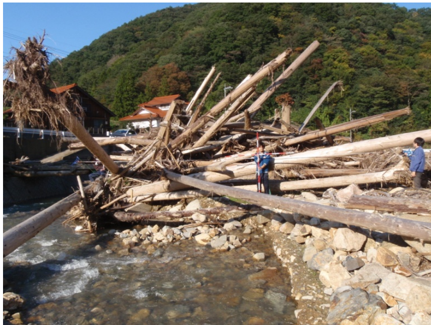
Figure 5.10 A back view of a woody debris jam at bridge without piers at Site 2 (taken from upstream of the river).
