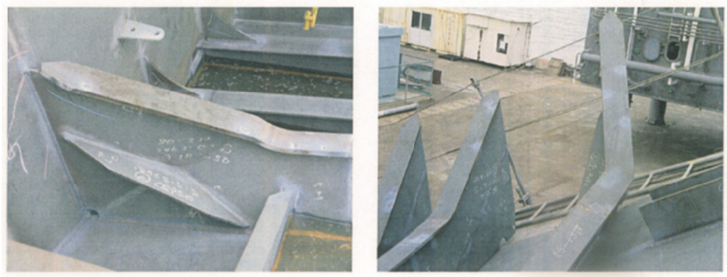
Fig. 1.3 Example of knuckled longitudinal stiffeners.
