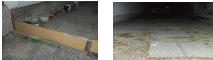
Fig. 4-25 & 4-26 Settlement of Planters and Difference of Pavement to State of Territory
