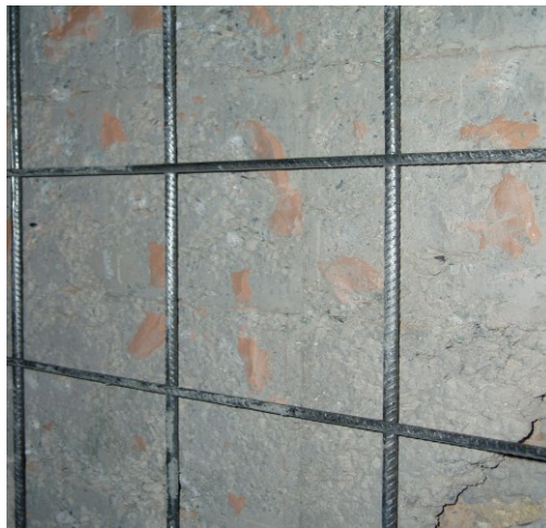
Figure 3.3 Steel wire mesh applied to the surface of URM wall
