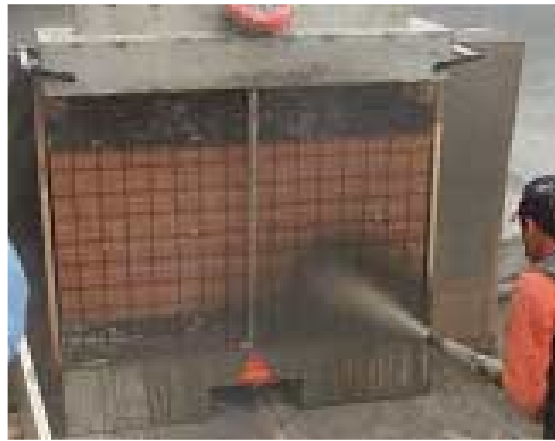
Figure 3.2 Externally retrofitted wall in shotcrete method [11]
