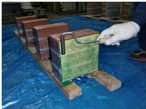
Figure 5.42 Removing air with roller
