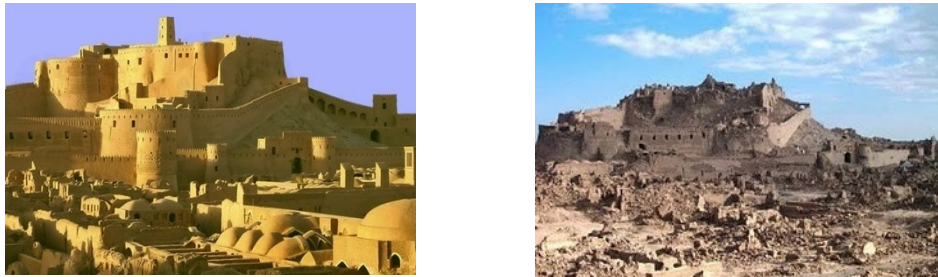
Figure 1.1 Bam historical masonry castle before and after 2003 Bam earthquake (Iran) [12]
