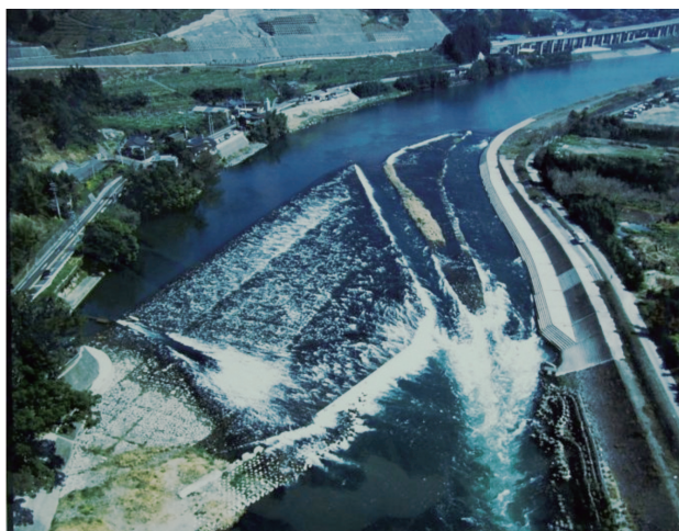
Fig. 5. Yamada diversion dam rehabilitated in 1980 (MLITJ, 2007).
