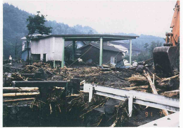
Fig. 11-4. A house broken by the debris flow of June 30 at the Yue River. (by Hirano, 2 July 1991 ).
