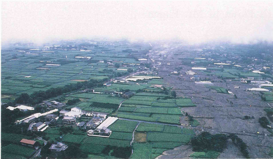
Fig. 11-1. Debris flow flooded into the protected low land on June 30. About 130 houses were broken. (by Hirano, July 2, 1991).
