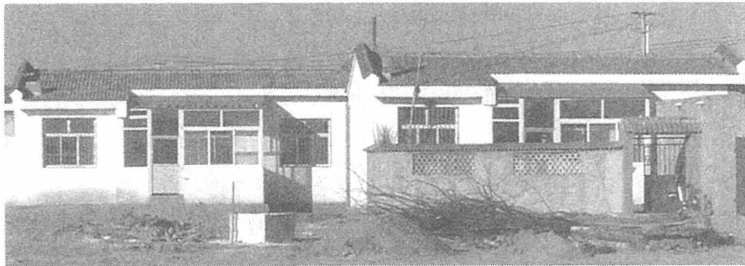
Fig. 4 Test object 2 – the new house
