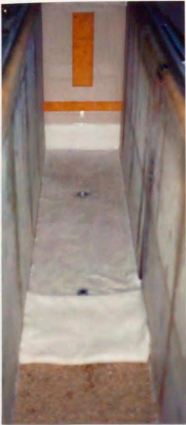
Photo. 6.4 Drainage layer, sand layer and nonwoven fabric
