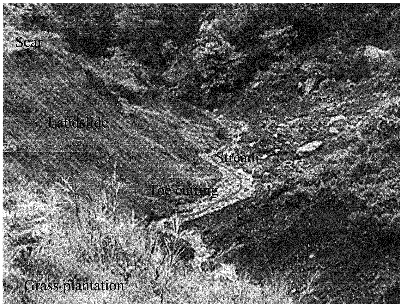
Photo. 1. Toe cutting of a deep seated landslide and side erosion by a stream in Parbat North watershed.
