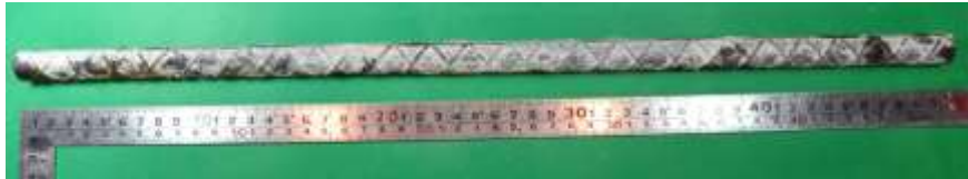
Photo 5.2 A 20-year-old deteriorated steel bar used in this study
