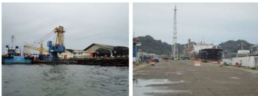
Photo 3.4 Existing load condition
