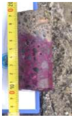
Photo 3.10 Phenolphthalein liquid spray at point 1
