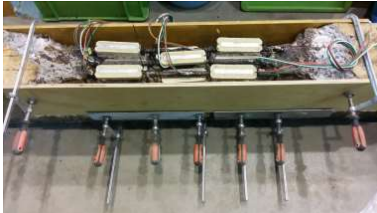
(a) Set up the formwork
