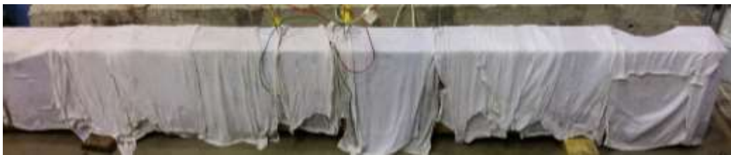
Photo 8.20 Exposure condition of RC beam under anode protection
