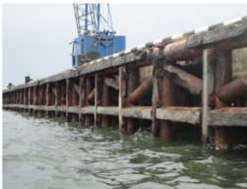
(a) Face fender structure
