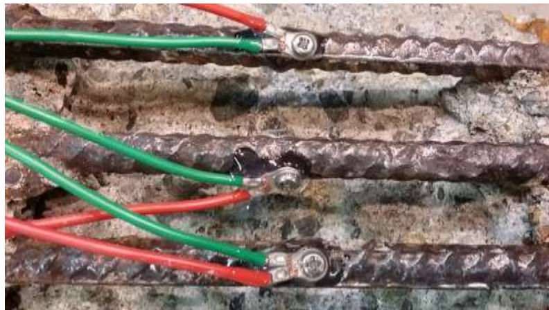
Photo 8.15 Step 4: protect the lead wire connection by epoxy
