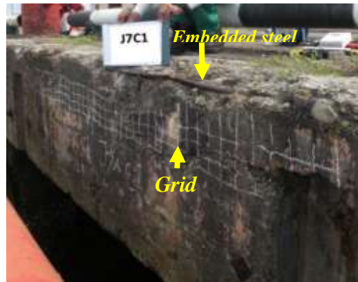
Photo 3.9 Preparation of grid system before half-cell potential measurement
