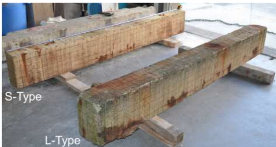
Photo 8.4 Appearance of beams over 40 years of exposure
