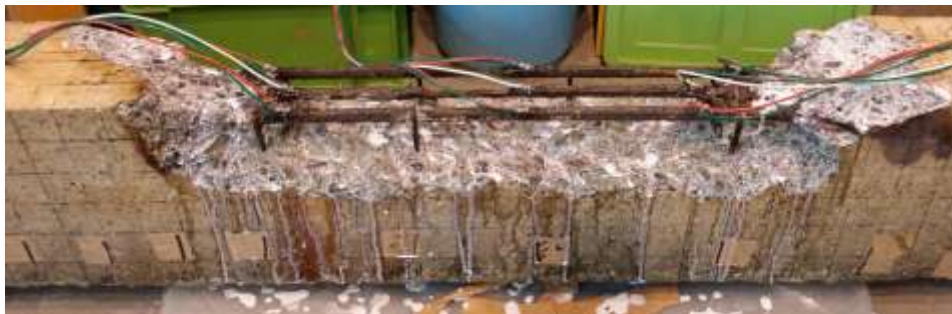
(b) Cover the repair area by RIS211E
