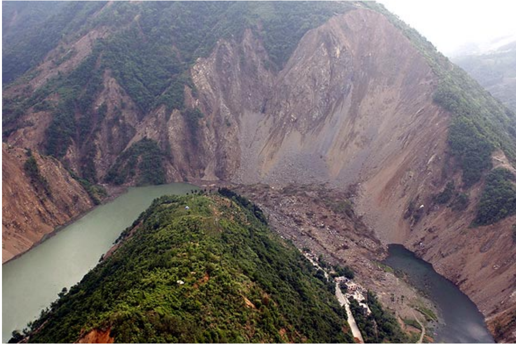
Figure 1. 2 Helicopter view of the artificial spillway in the Tangjiashan landslide dam (adopted from Xinhua News Agency)
