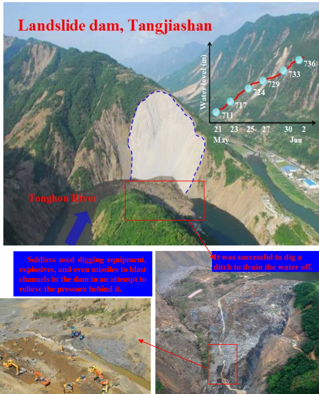
Fig 1.9. The Tangjiashan landslide dam and its discharge channel (Tang et al., 2009; Liu et al., 2010; Chen et al., 2011.)
